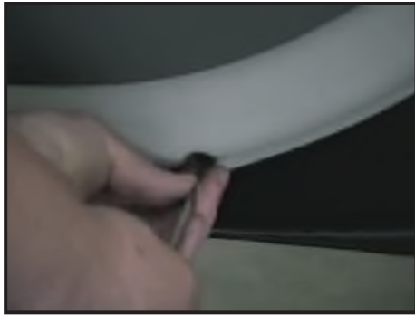
19. Remove screw from lower right of panel.
